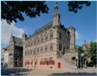
10 Deventer Weighing house - 1531 (p. 44-45)
