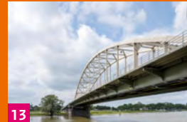
13 The Wilhelmina bridge over the IJssel, at Deventer. (p 28)
