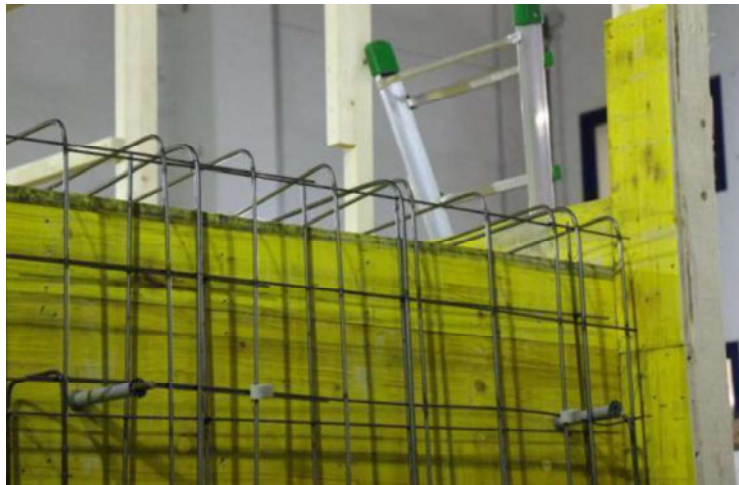
Figure A.8: Detail of the in-floor bent rebars placed in a wall-slab joint of the EUC-BUILD-3 specimen (adapted from [Brunesi et al, 2017]).
