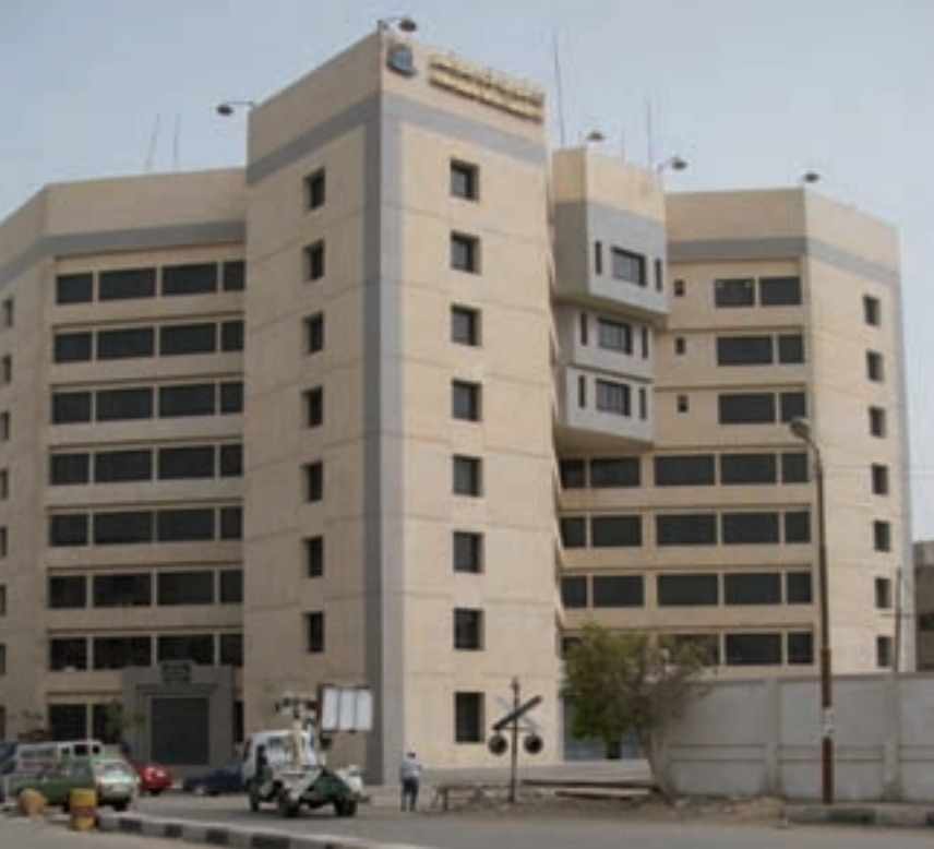
Main office FADWASC
