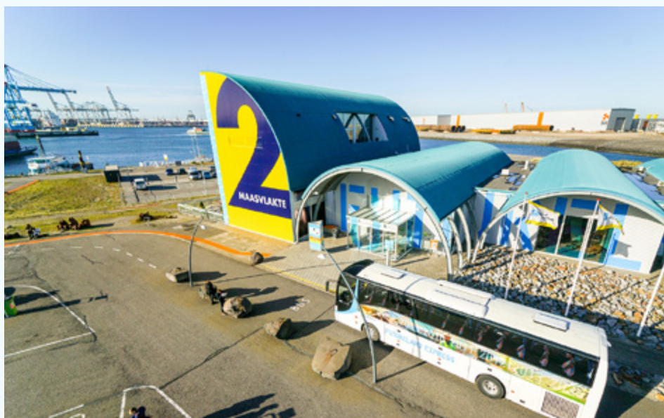
FutureLand (BRON: DUTCH DRONE COMPANY/HBR)
