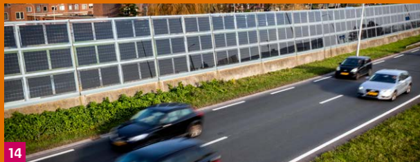
The provincial road between Delft and Zoetermeer is the first road with a closed energy system. The solar panels on the noise barriers provide sufficient energy for the lighting along the road. (p. 17)
