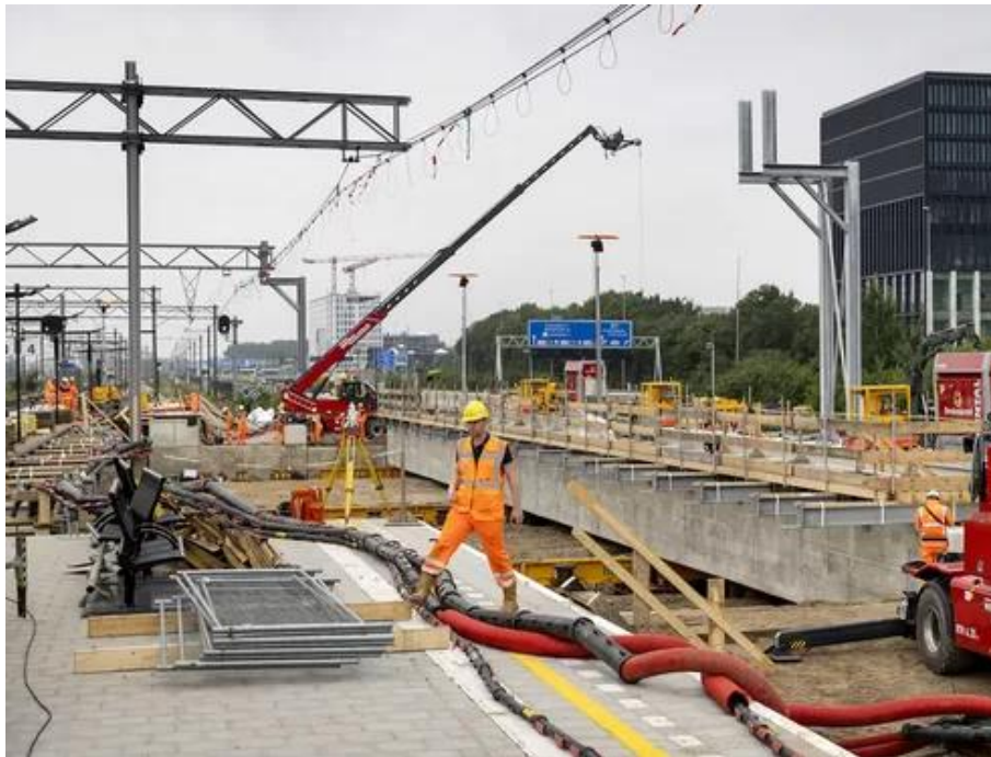
Dakdelen Brittenpassage Station Amsterdam-Zuid
