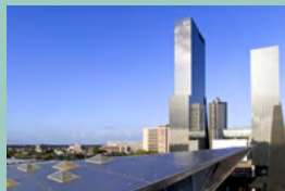
Solar panels at the roof of Rotterdam Central Station (p 3)
