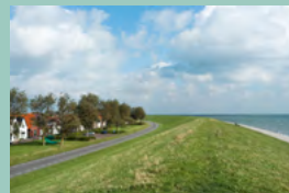
Reinforcing the dikes on the island of Texel to protect the village of Oudeschild (p 12)
