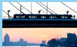
Tram crosses Erasmus Bridge in Rotterdam while water taxi passes below. (p 31)
