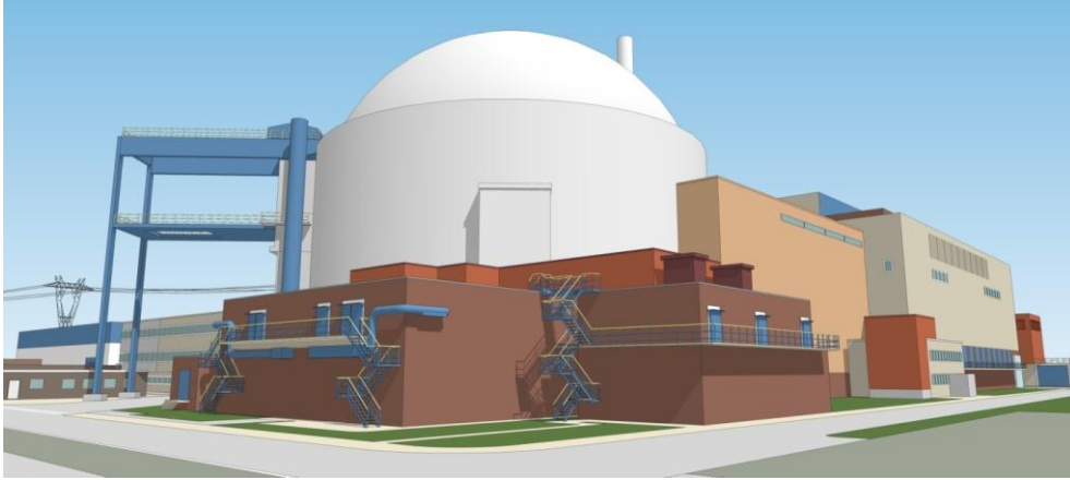
Figure 1.4 Borssele Nuclear Power Plant
