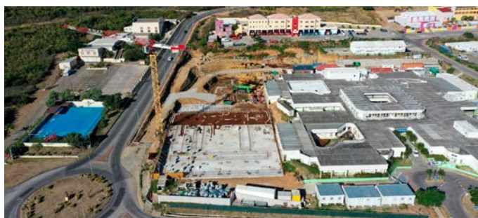
Construction of the hospital
