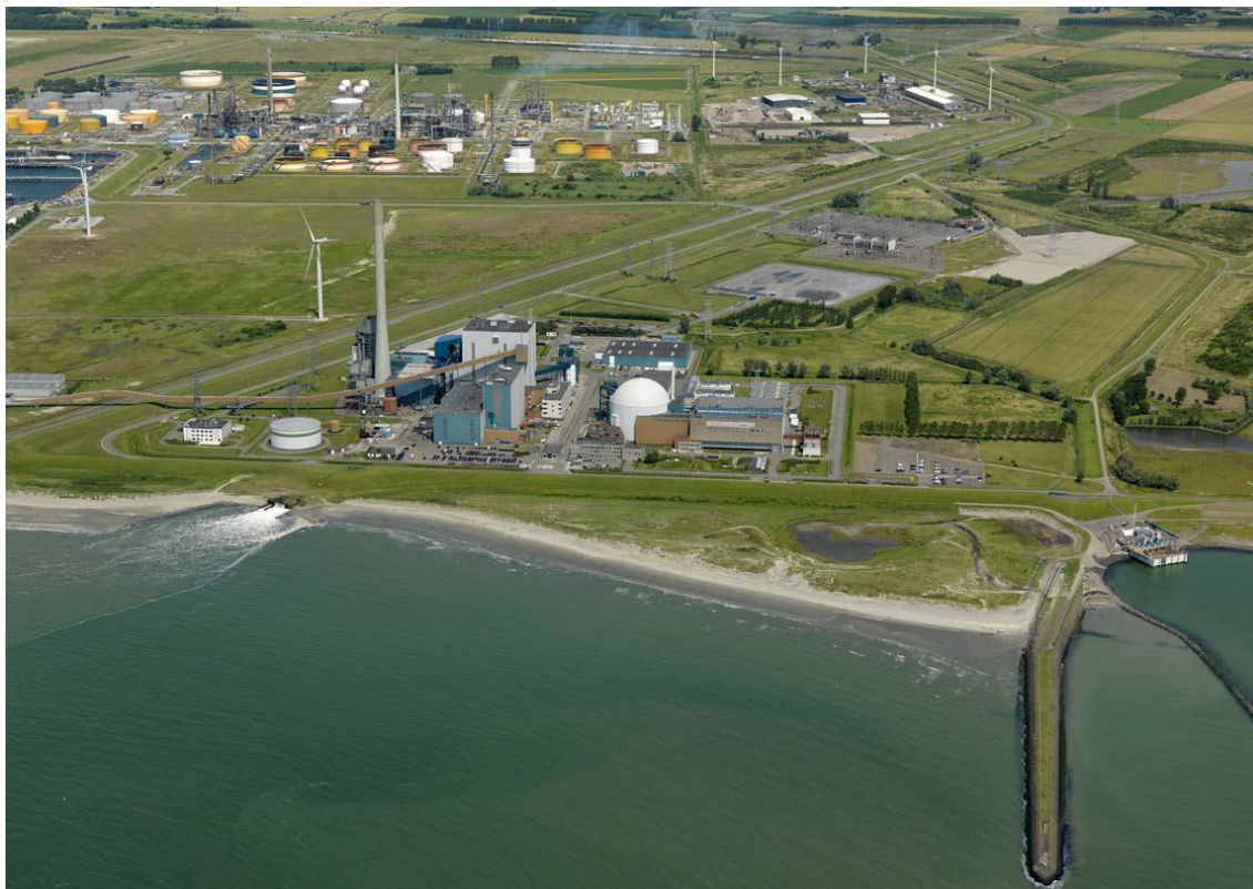
Figure 1-2 Aerial photograph of EPZ site. Front middle: the NPP, and left of it the coal-fired unit. Front left: outlet coolant, front right: intake coolant. Behind the EPZ site: industrial area.
