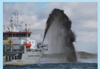
12 Zandsuppletie kust (sand supplement in front of the coast) Walcheren (p. 41)
