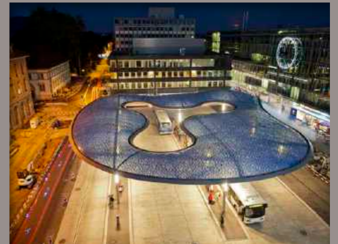
4. Aarau Bus Station canopy
