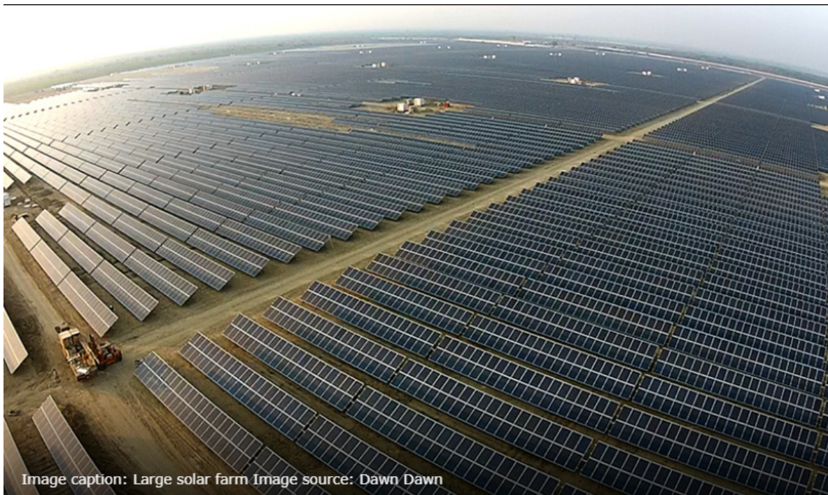
Figuur 25 Zonneparklandschap in Pakistan (Bron: https://www.masterbuilder.co.in/pakistan-setting-worlds-largest-solar-park/ ).
