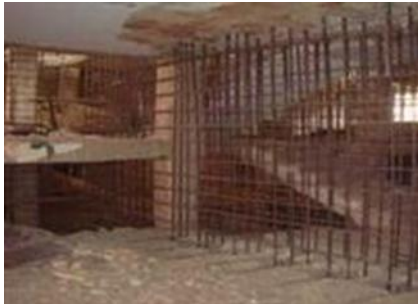
Figure 40 Replacing existing masonry walls with reinforced concrete walls.
