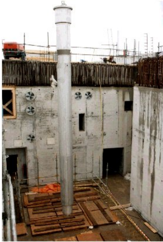
Figure A.4. Emplacement of the wells during construction.
