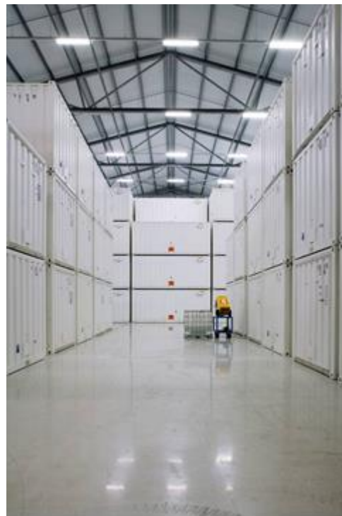
Figure A.3 The storage of radioactive calcinate from phosphor production in the COG
