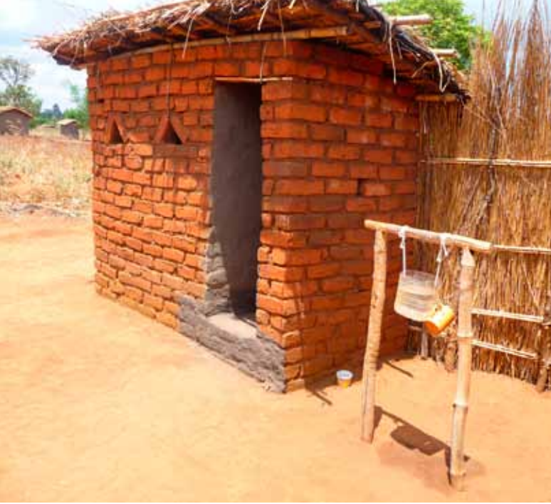
Latrine with handwashing facility
