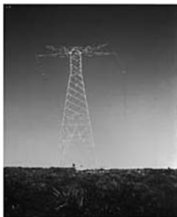
Photo 11 Self-supporting 600 kV tower
