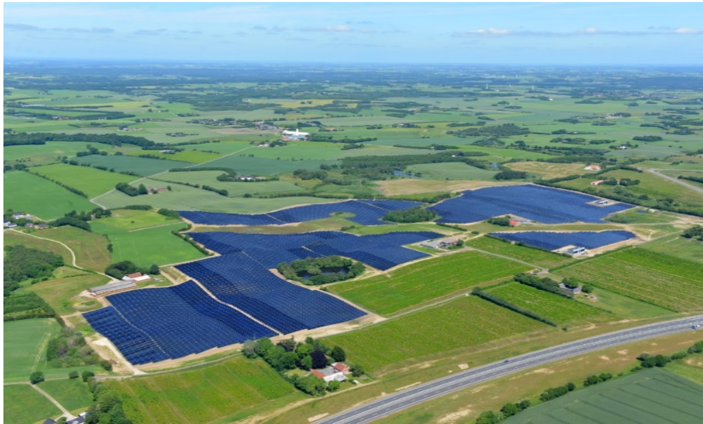
Figure 5.3 - Sejling Hede sun heat plant for district heating developed and owned by Silkeborg utility
