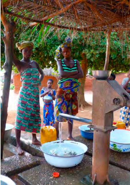
Borgou; protected well with handpump
